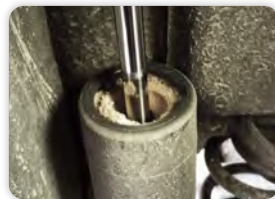
Broken bump stop
