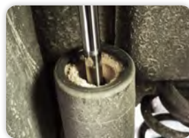
Broken bump stop
